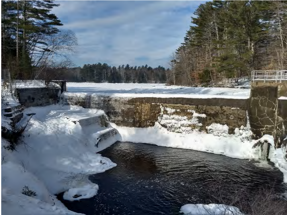
Photo No. 13 – Upper Dam – Downstream side of dam. Note right abutment training wall and concrete apron.
