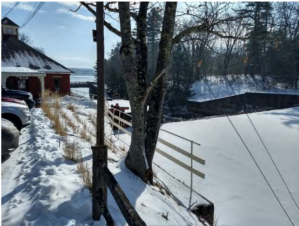
Photo No. 16 – Lower Dam – Upstream side of Left Abutment, looking downstream.
