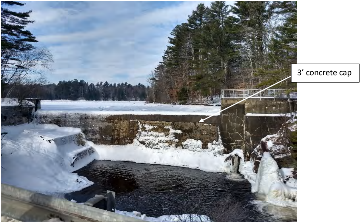
Photo No. 3 – Upper Dam – Downstream face. Note 18” and 8” outlets flowing.
