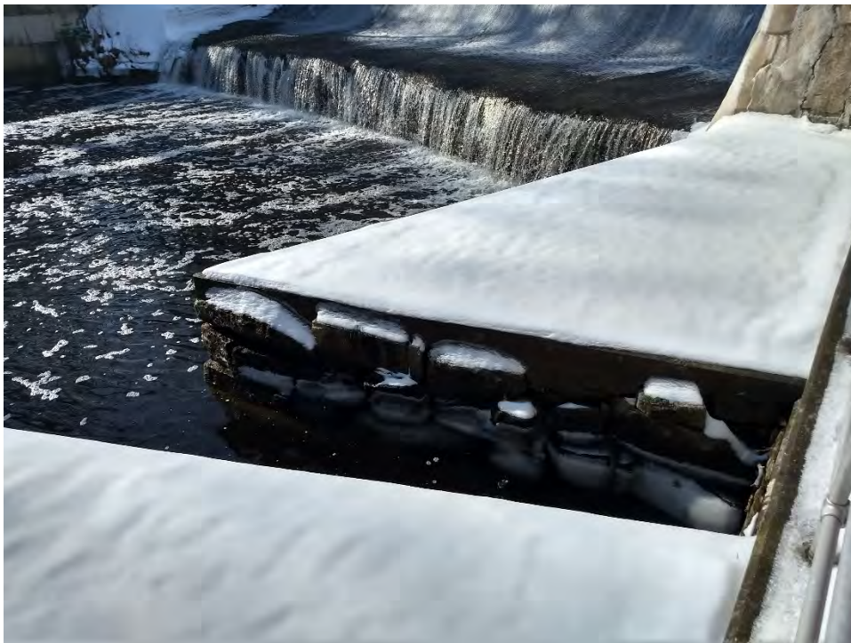
Photo No. 20 – Lower Dam – Downstream masonry training wall on left side.
