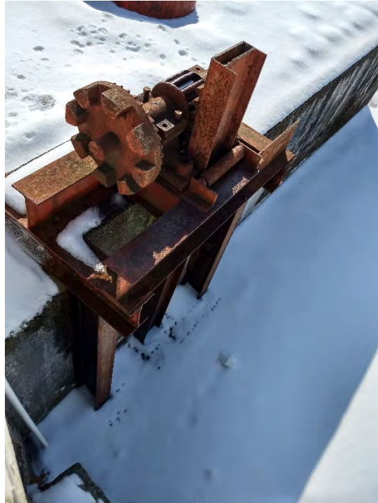
Photo No. 17 – Lower Dam – Intake on left abutment.
